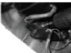
(2) Remove two screws on comp base
