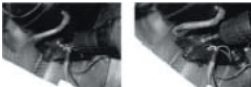
(2) Loosen two screws on comp base
