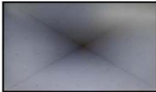
Abnormal Power Section
